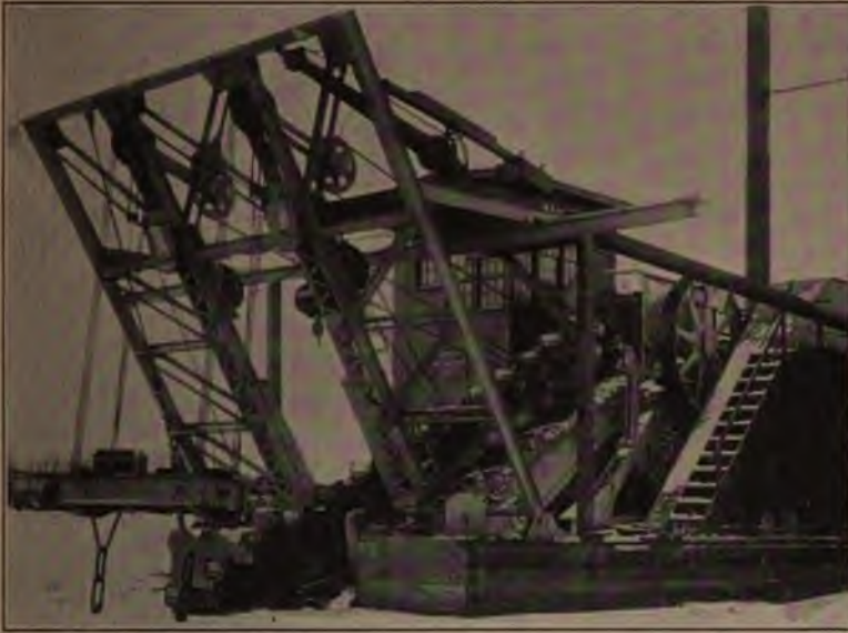
View of Front End of Ladder Dredge on New York State Barge Canal. Figure 94.
